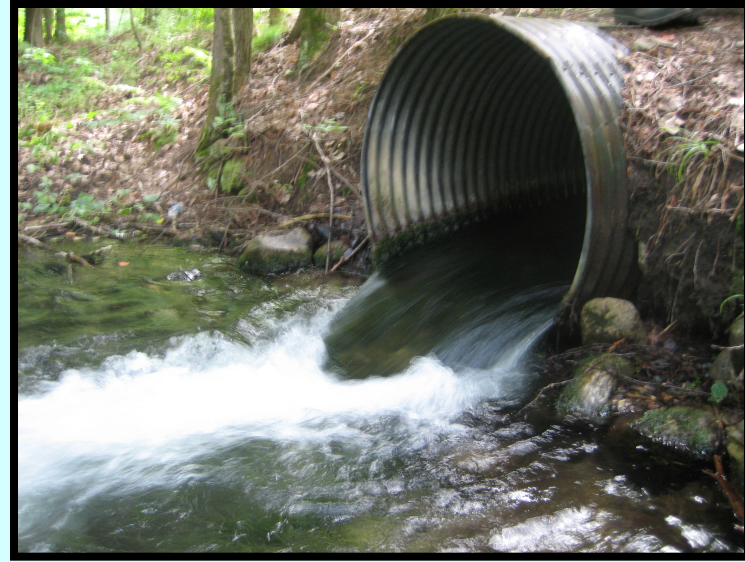
Finch Creek east outlet at Elder Road
