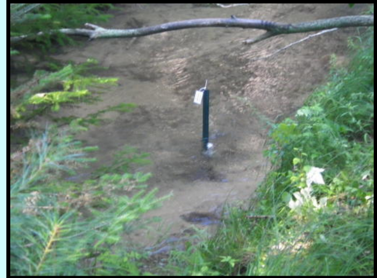
Completed installation in Shanty Creek
